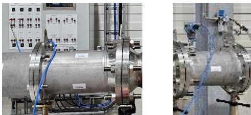
Picture 2 connecting pipe spools.
